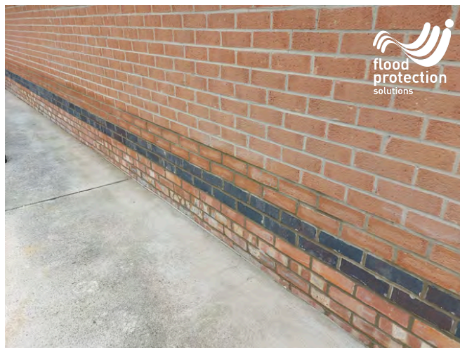
Repointed with waterproof additive; curing in progress
